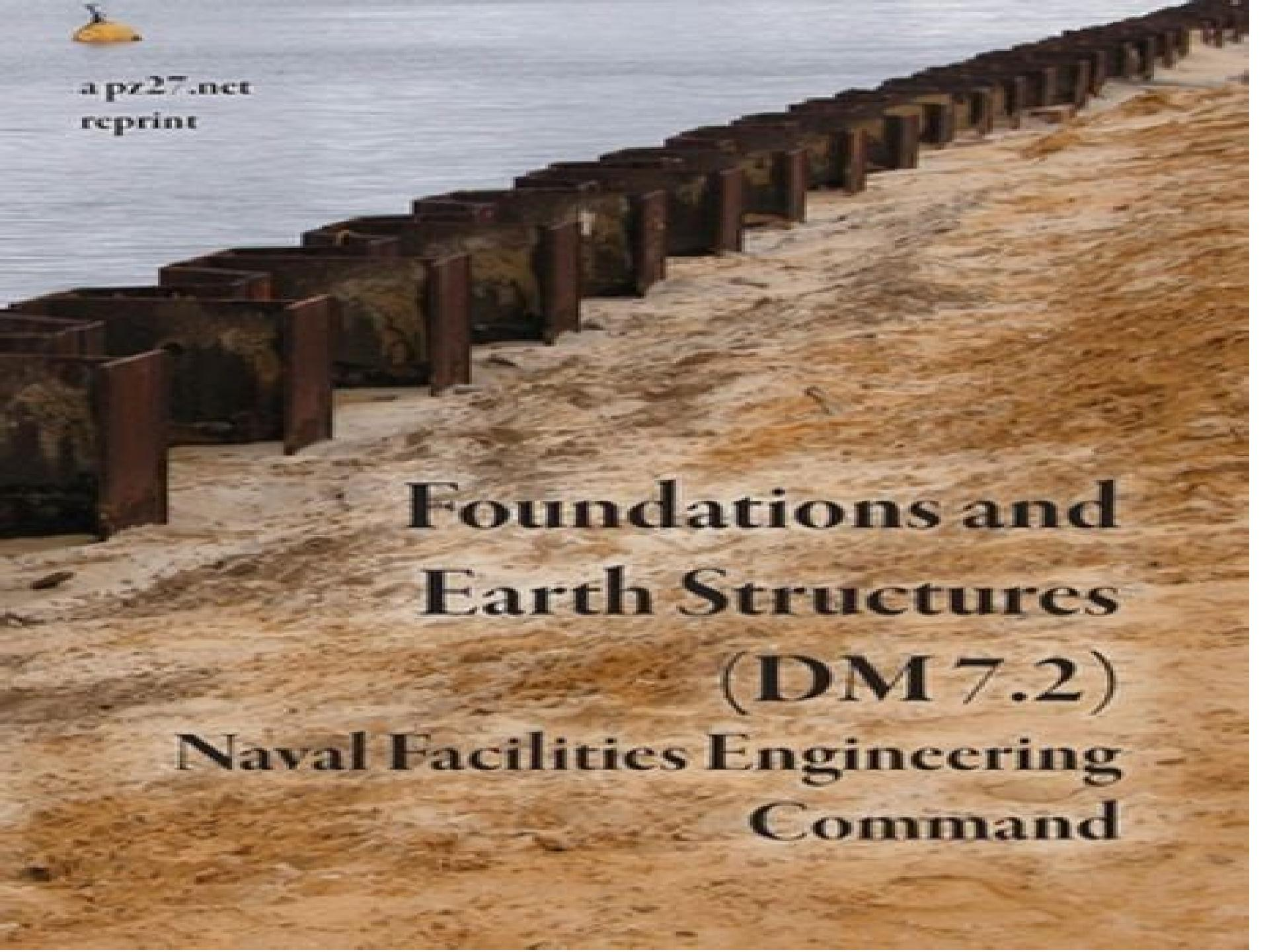
The background image shows a coastal erosion control structure. It consists of a series of vertical sheet piles driven into the ground, with a sand berm or embankment built up behind them. The ground appears to be sandy and eroded. The ocean is visible in the background.
